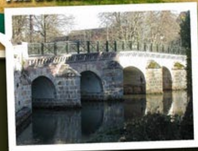
THE GUILLERIE BRIDGE
